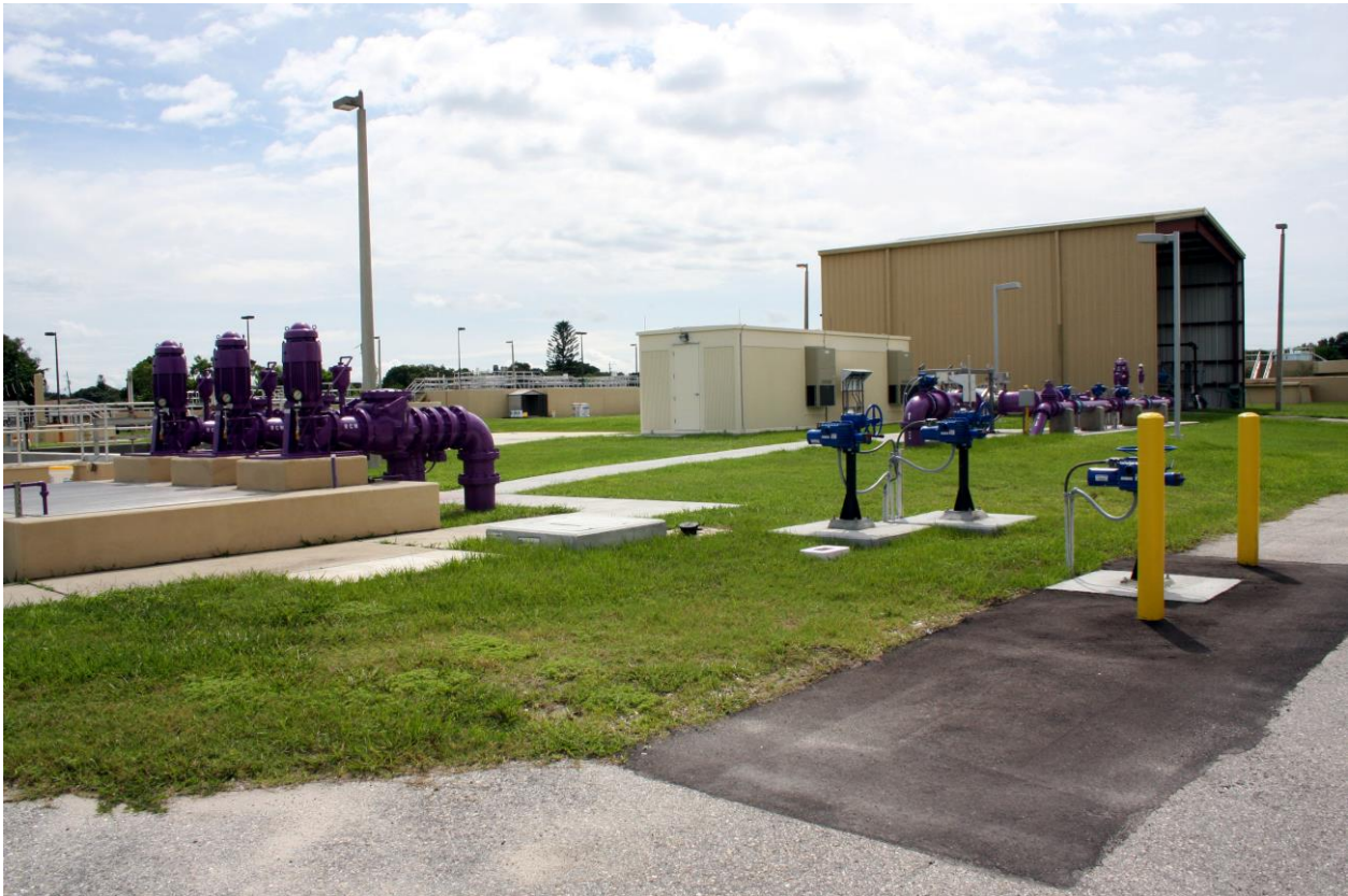
The Wastewater Treatment Plant processes water, sewage and reclaimed water for public purposes.
